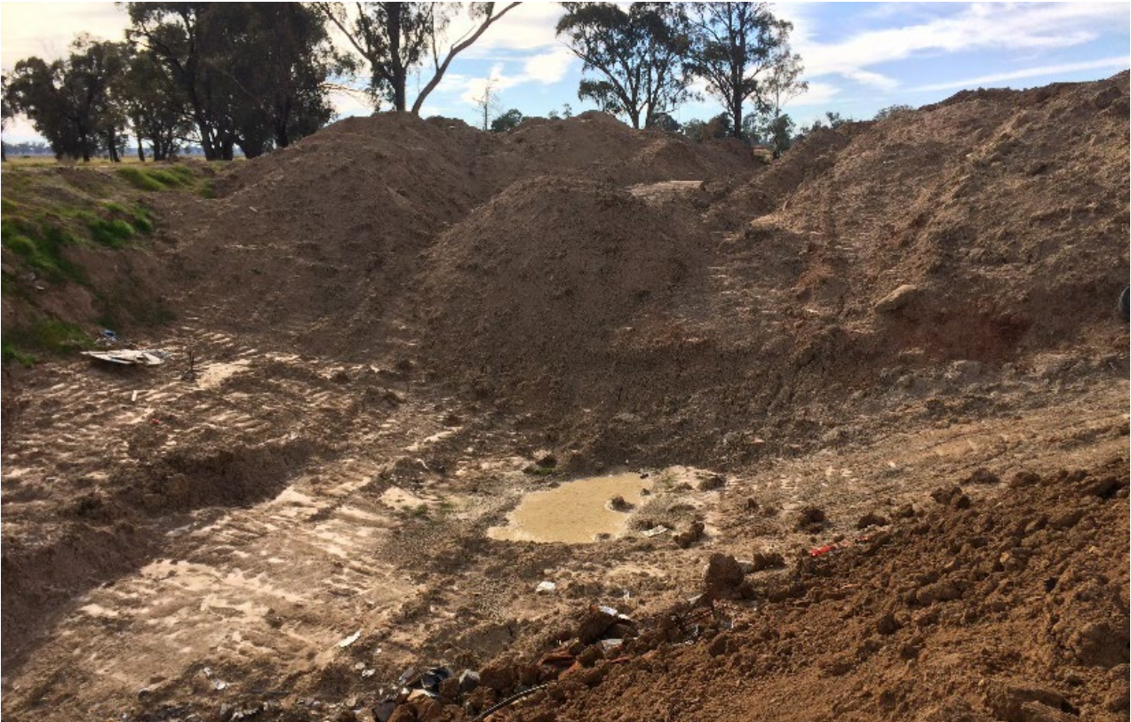
Figure 2-3 Excavated waste cell.
