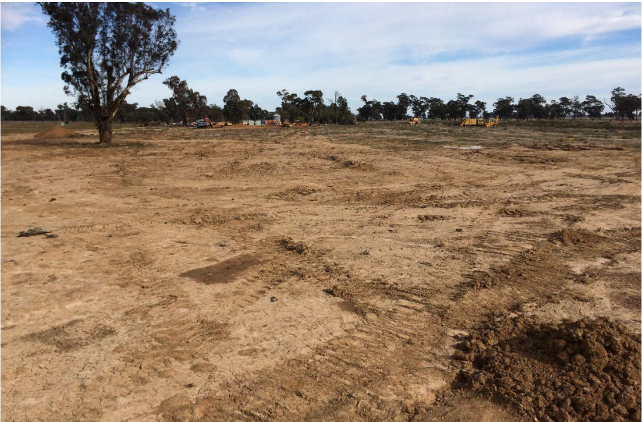
Figure 2-5 Filled and capped waste cell.
